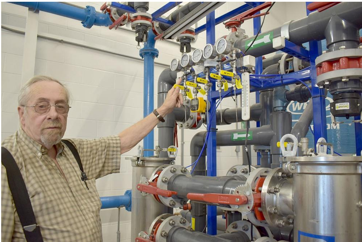
Lanagan Mayor Stan Haywood indicates where pressures on the filtration vessel are measured by gauges at the new water treatment plant.
